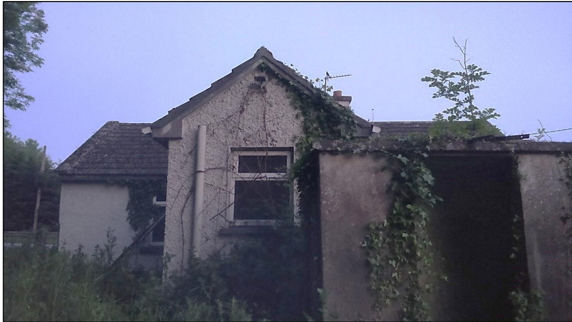
Plate 4-1 Ivy Cover at Rear of Identified Roost
